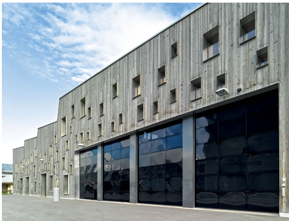
TOP. ALR F42 Vitraplan with grey tinted glazing integrated in the glass facade
