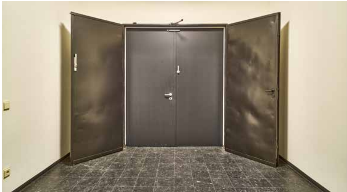
The historic sheet steel door has been preserved and joined by a fire-rated door to form a double door system.
