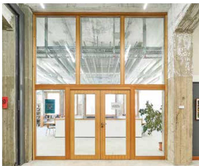
Horizontal view of acoustic-rated fixed glazing with integrated door.
