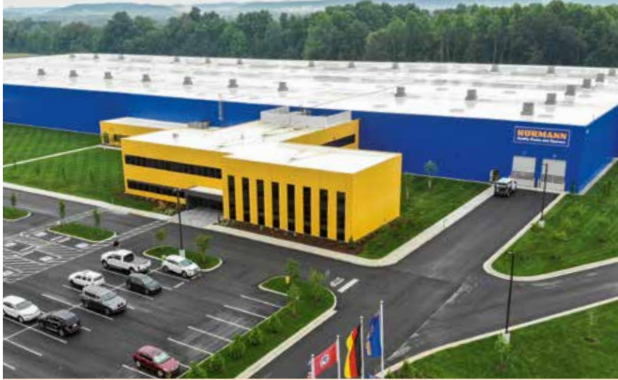
The new production location in Sparta, Tennessee, USA, was completed in October 2020.
