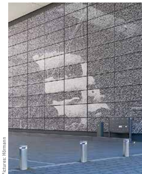
The bollards integrate into the architecture.
