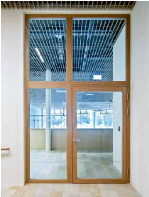
Transparency thanks to storey-high glazing.
