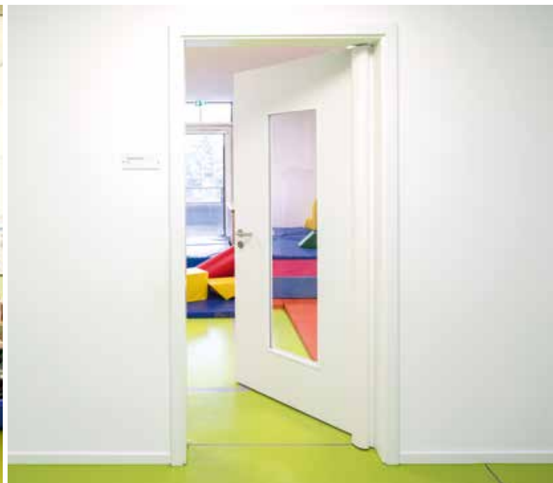
Finger protection rollers are designed in white to keep them as subtle as possible. A glazing cut-out shows the children who is behind the door.
