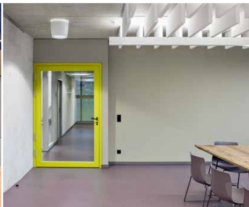
Several doors have excess widths and are therefore fitted to four hinges.
